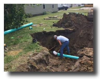
The City of Sullivan was experiencing large amounts of infiltration resulting in raw untreated sewer backing up into homes and other areas within the City. It was determined that the Sewer and Collection System installed in the 1930's had outlived its useful life and failed, resulting in infiltration from cracked or collapsed sewer pipes.
