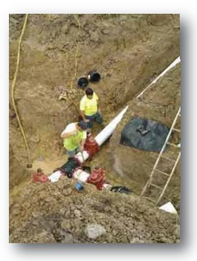
This project consists of approximately 4,500 lineal feet of 10" PVC water main extension to serve future development sites. Milano & Grunloh Engineers assisted in obtaining funds, surveying, design and construction inspection for the project.
