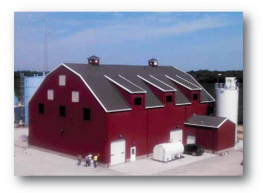
The Gila Water Treatment Plant is EJ Water Cooperative, Inc.'s second water treatment plant in the past five years. The water treatment plant has a capacity of 1.5 MGD and a 1 MGD ground storage tank. Milano & Grunloh Engineers, LLC assisted with obtaining funds, surveying, design, and construction inspection. The plant started providing water in the fall of 2015. The project was funded with Department of Commerce and Economic Opportunities and USDA Rural Development funds.
