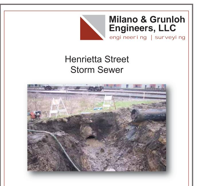
Milano and Grunloh worked with the City of Effingham to design and construct the Henrietta Street Storm Sewer, consisting of 1500 feet of 36" Storm Sewer, including boring 371 feet of 48" Steel Casing under the Railroad Right-of-Way and Illinois Route 40. Milano and Grunloh assisted in obtaining the necessary permits from the Railroad and State of Illinois. The cost of the Project was \$367,000.
