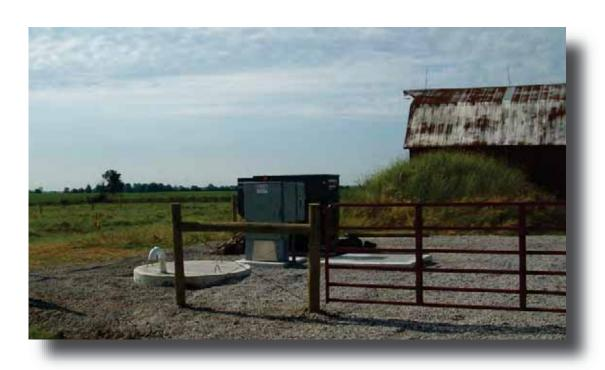
The Village of St. Peter was experiencing large of amounts of infiltration, sewer backups, and a failing lift station that needed replaced. The Village secured a \$44,500 design grant, \$182,000 in USDA Rural Development funding, and a \$350,000 DCEO construction grant. The project replaced the failing lift station and 2,500 lineal feet of sewer main.
