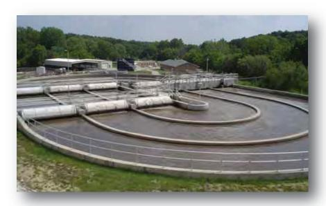
This project consists of major improvements to the City of Effingham waste water treatment facilities. The improvements included a new screen, new grit collection equipment, a new activated sludge oxidation ditch, new secondary clarifier equipment, a new return sludge pumping station, new sludge transfer pumps, anaerobic digester improvements, new sludge storage tank, and all piping, fittings, site work, excavation, backfill, electrical work and demolition.
