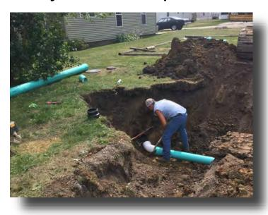
The City of Sullivan was experiencing large amounts of infiltration resulting in raw untreated sewer backing up into homes and other areas within the City. It was determined that the Sewer and Collection System installed in the 1930's had outlived its useful life and failed, resulting in infiltration from cracked or collapsed sewer pipes.
