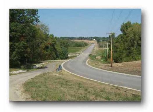
Phase 1 of Evergreen Avenue consists of a 6,946 foot extension of Evergreen West of Effingham. Milano & Grunloh Engineers furnished the environmental report, preliminary and final engineering study and Right-of-Way on Evergreen West along with material testing, staking and construction inspection on parts of the road.
