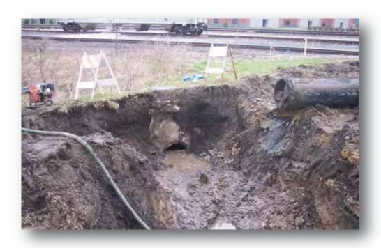
Milano and Grunloh worked with the City of Effingham to design and construct the Henrietta Street Storm Sewer, consisting of 1500 feet of 36" Storm Sewer, including boring 371 feet of 48" Steel Casing under the Railroad Right-of-Way and Illinois Route 40. Milano and Grunloh assisted in obtaining the necessary permits from the Railroad and State of Illinois. The cost of the Project was \$367,000.
