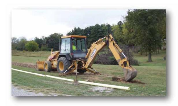
The Village of Watson serves approximately 300 users with 70,000 linear foot of watermain. The Village was experiencing water main breaks and low pressure due to the aging cast iron watermains within their system. Milano & Grunloh Engineers, LLC worked with the Village to develop project areas for the proposed improvements, completed all permitting, applying for grants and loans, and all of the engineering and surveying for the project.
