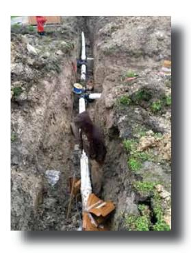
In 2012, the Village of Stewardson successfully applied for a \$350,000 DCEO Public Infrastructure Grant. The Grant monies along with bank loan funds of \$350,000 as leverage, allowed the Village to replace 26,000 lineal feet of seriously deteriorated and undersized ductile iron watermain. The replacement of the watermain succeeded in alleviating the health risk to 194 households and 453 person living in the West half of the Village.
